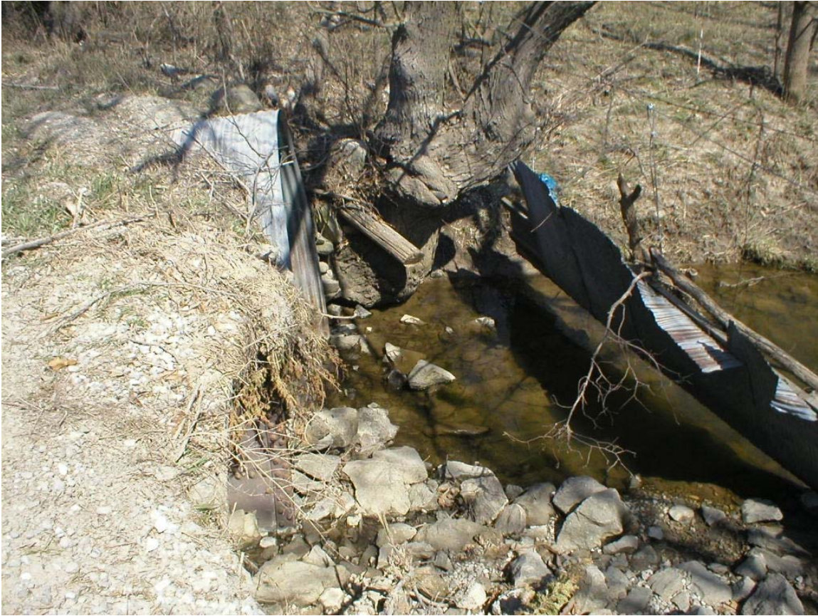
Photo 10.3-vi Remove Farm Fences Obstructing Channels
