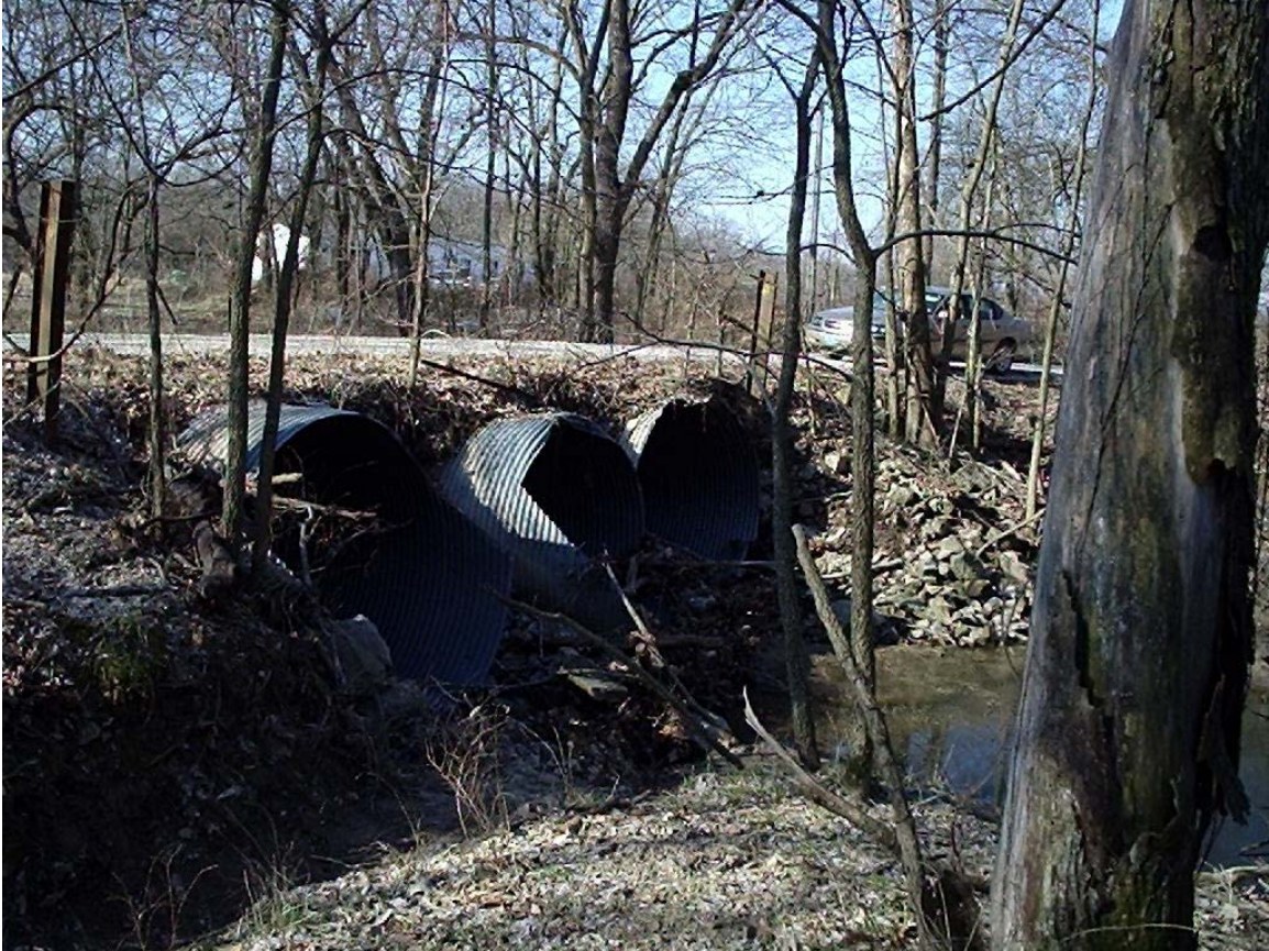
Photo 10.3-vii Reshape Culverts
