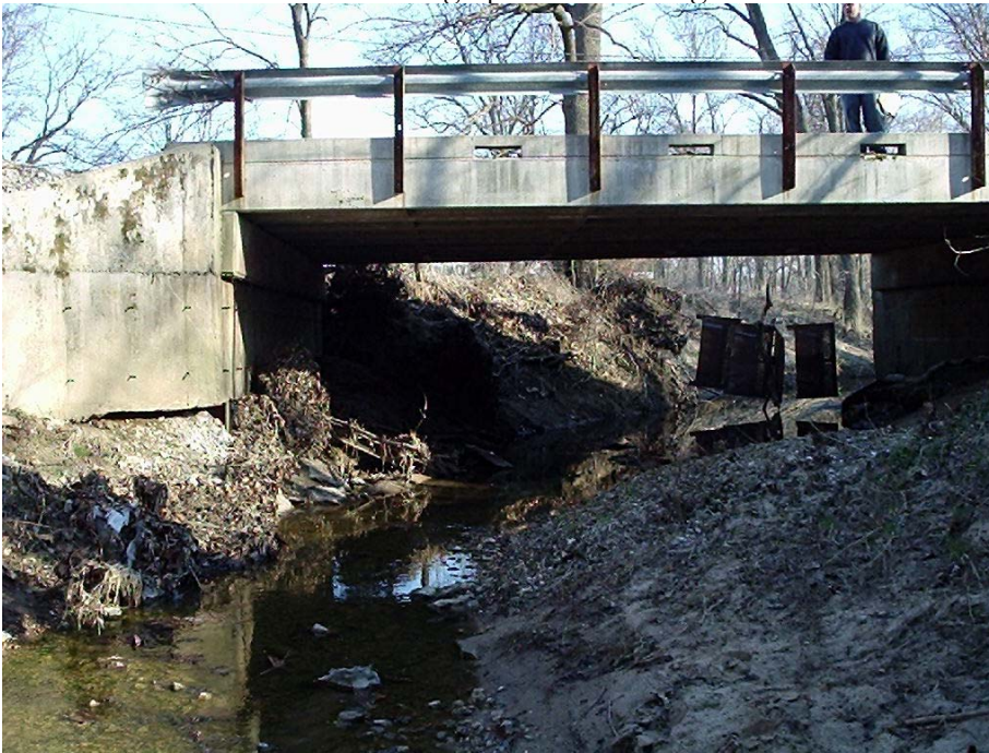
Photo 8B. Gans North. Looking upstream at bridge.
