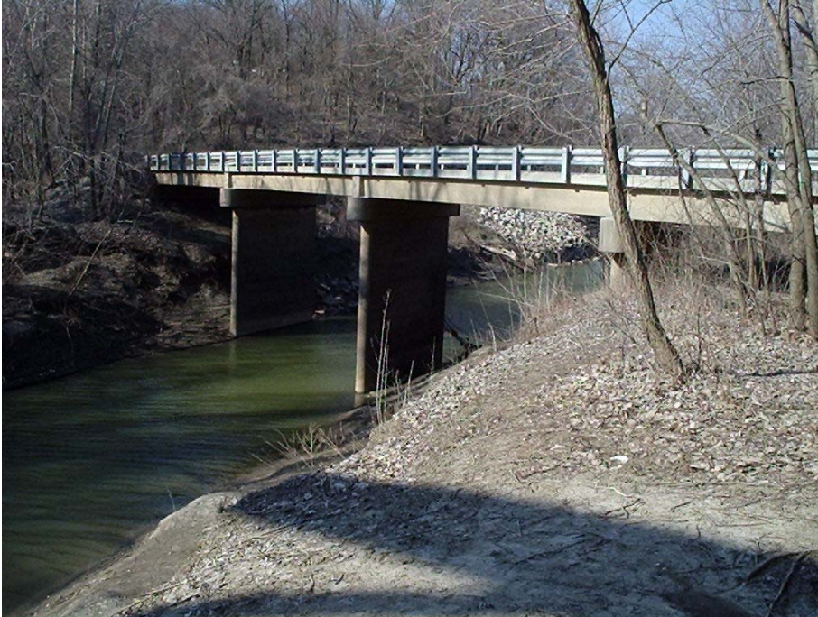
Photo 13D. Mayham Branch. Bridge.
