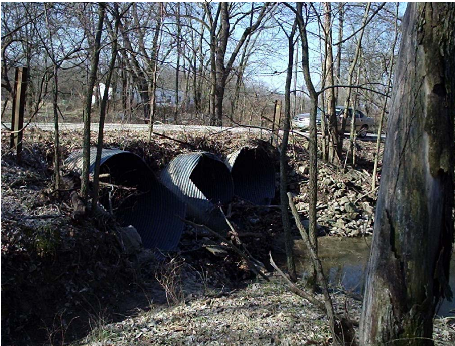
Photo 10B. Gans South. Looking downstream at culvert.
