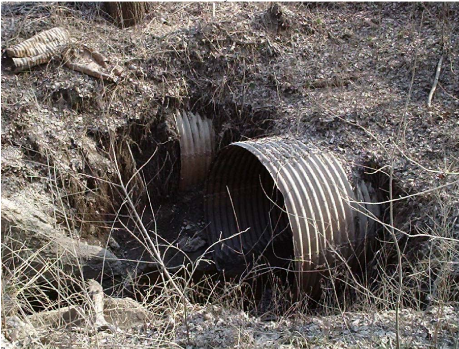
Photo 12B Missouri River Tributary. Buried culvert.
