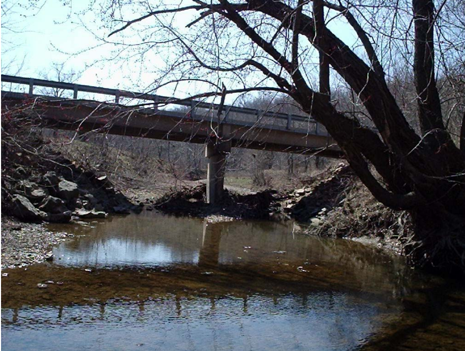
Photo 7B. Fox Hollow Branch. Looking upstream at bridge.
