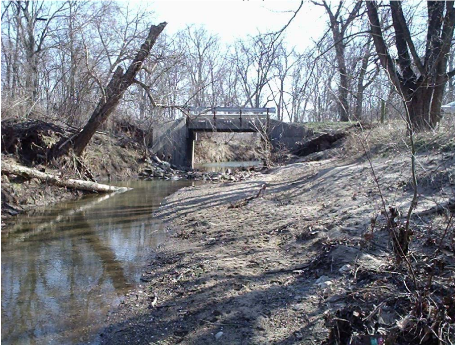
Photo 9B. Gans Main Branch. Looking upstream at bridge.
