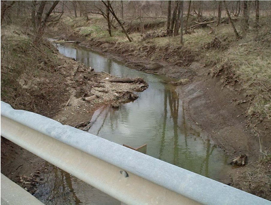
Photo 1A. N. Branch Little Bonne Femme from the bridge. Looking downstream.
